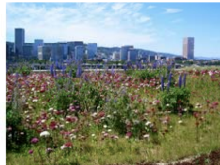
Multnomah County Building ecoroof
